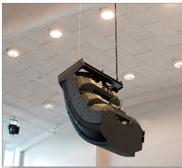
Three array speakers per side over five meters up in the air, plus four subwoofers on the floor.
